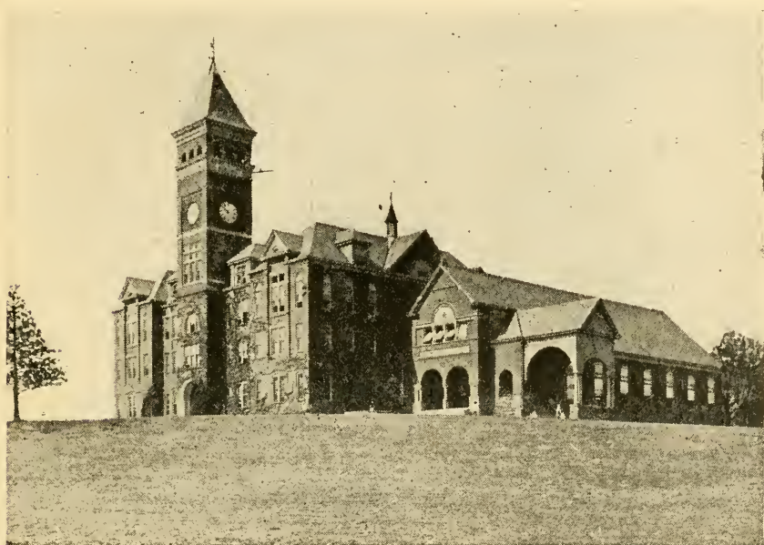
Administration Building at Clemson College.
